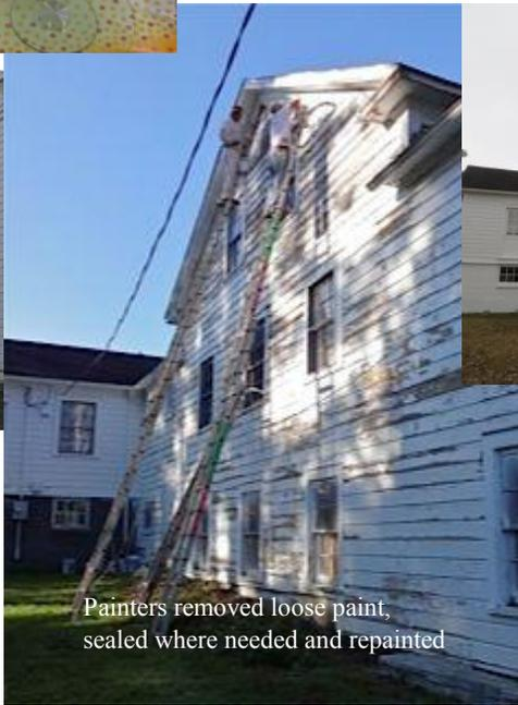
Painters removed loose paint, sealed where needed and repainted
