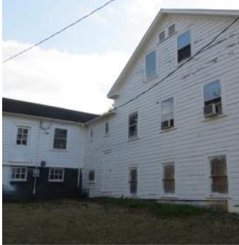
The LFR Building, like the Church, had missing and loose paint allowing moisture to penetrate our wood.
